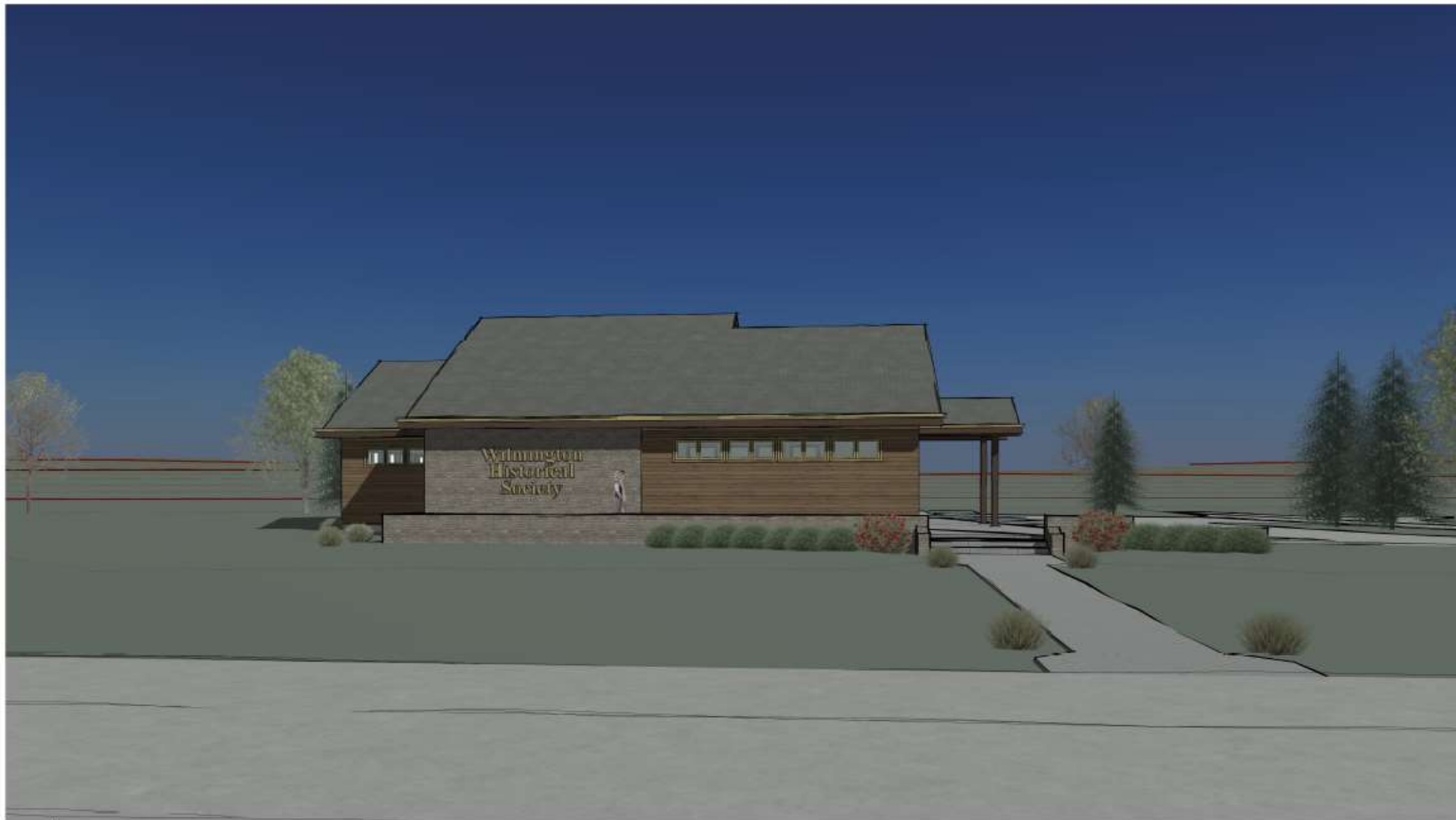
1 VIEW TO NORTHWEST SS-2
